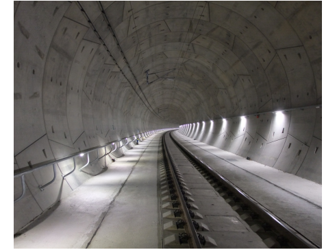
Tunnel Ejovice, CZ 2019, CZ
